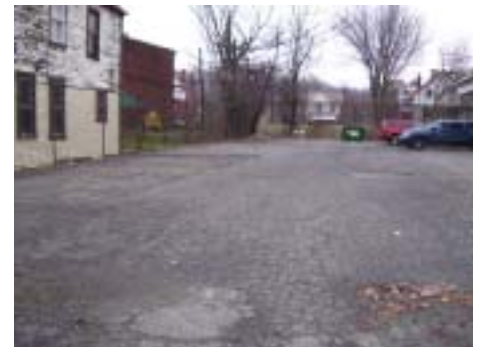
The building and the grounds are in deplorable condition but Unity Community Lutheran Mission continue to be a beacon shining the Gospel in the Homewood-Brushton area of Pittsburgh. For each day that progress on the new building is not made, the current site continues to use valuable resources just to keep the walls up.
