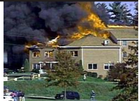
As board members and congregational delegates were traveling to the annual meeting on Sunday, November 5, 16 fire companies were battling the blaze on the roof of Haven I.
